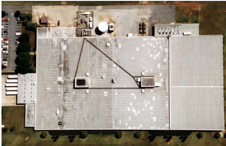
Figure 6. Photograph of a flat roof.
