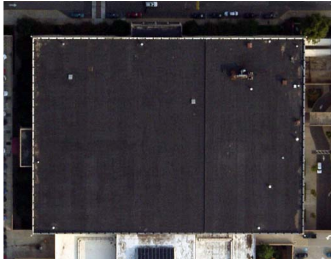
Figure 4b) Thermograph of a roof.
