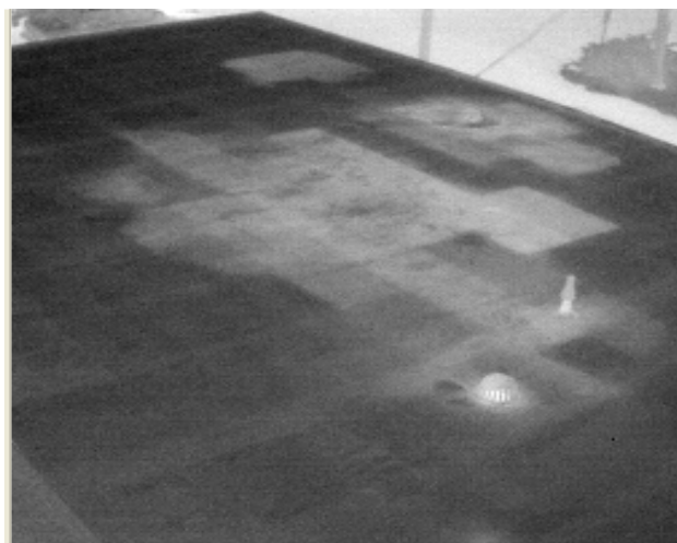
Figure 2) On-roof IR image.
