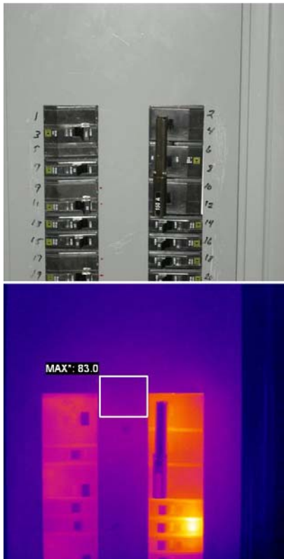
.Figure 2 – Visual and thermal image of a panel with covers on.
