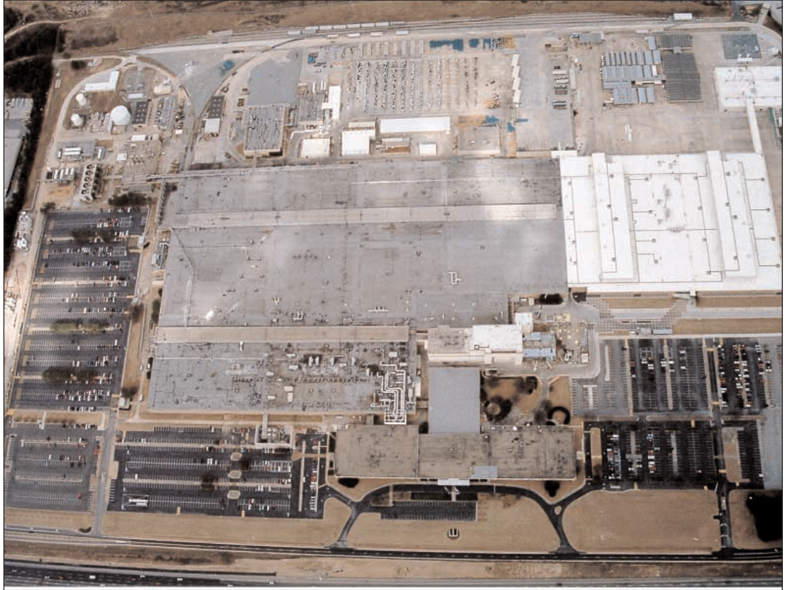
Figure 3: Aerial photograph of a 2.2 million sq.ft. building that took 25 minutes to infrared survey from the air. We calculate a crew of three would have taken 5–7 nights to infrared survey from the roof.
